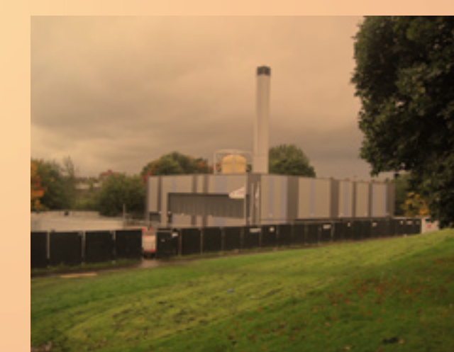
DH pipes before being laid in Edinburgh Wyndford energy centre, Glasgow
