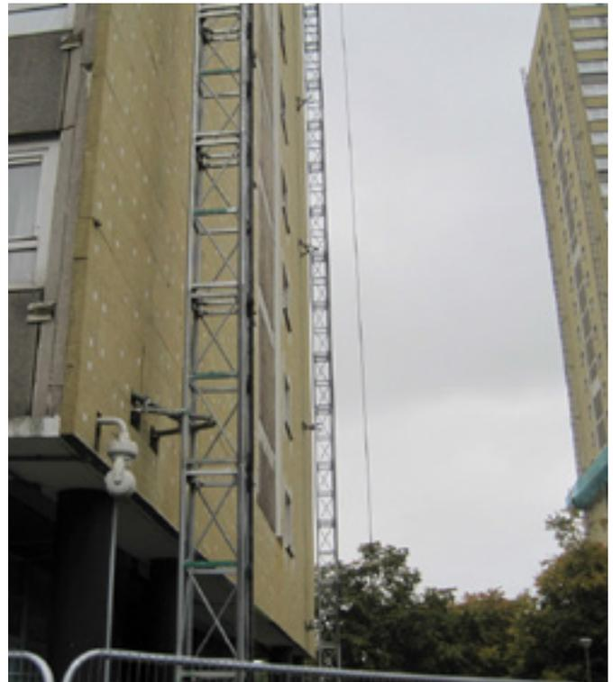
Tower blocks in Glasgow being fitted with external insulation.
